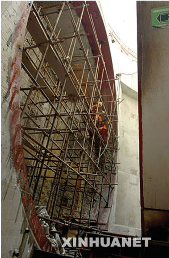
Fig. 85.4 Workers constructing part of the tunnel to cross under the Yellow river. (Source: Changjiang (Yangtze) Water Resources Network at www.cjw.gov.cn/news/detail/20070508/91050.asp . Xinhua News Agency Photo)
