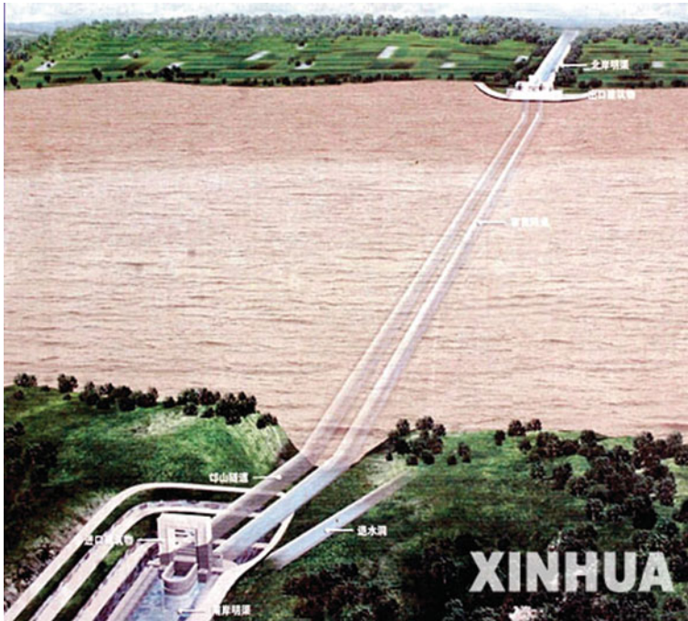
Fig. 85.3 Artist's rendering of parallel tunnels crossing underneath the Yellow river. Similar tunnels will also be part of the central route. (Source: Changjiang (Yangtze) Water Resources Network at http://www.cjw.gov.cn/news/detail/20070508/91050.asp . Xinhua News Agency Photo)
