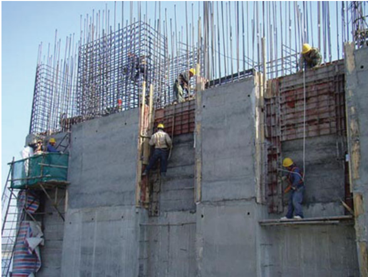
Fig. 85.5 Workers increasing the height of the Danjiangkou Dam in 2008. (Source: South-North Water Diversion website at http://www.nsb.gov.cn/nsbdgc/zxgc/djk/20080313/200803130017.htm )
